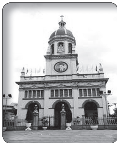
Figure 3 the Santa Cruz Church (the present building)
